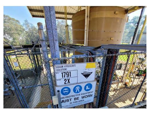
Isolation, Decommissioning, removal offsite and safe & good 4 off Existing Sodium Hypochlorite dosing pumps, and associated piping, valves and inline equipment and replacement with new like for like commissioning and handover to SW. All piping was double containment PE electrofusion. AJM United have electrofusion welding machines and experienced trained, ticketed welders.
