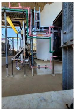
Working with chemical systems is always high risk and challenging, on this project AJM United had to plan to detail, ensuring that the existing assets are not disturb eliminating or reducing to very unlikely any possibility of hindrance to the plant and or Sodium Hydroxide plantation. The works included decommissioning, removal and disposal of old and installation of new dosing skids and tanks, steel supports, double containment piping in UPVC materials, valve and all inline equipment.
